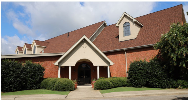
Church from parking lot. Entry Portico is at center. Right dormer is in the upstairs multi- purpose room. The three dormers to the left side are in the Sanctuary.
